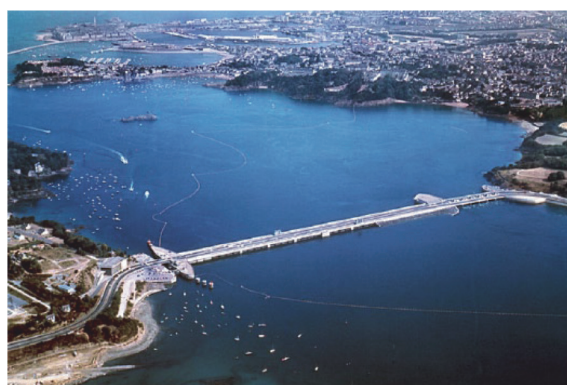
La Rance tidal barrage (above) in northern France has generated electricity since 1966, and repaid its construction costs in 20 years. Its electricity costs just € 0.12 (11p) per kWh.
